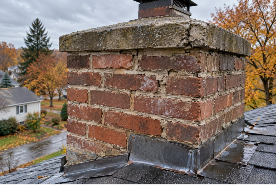
Original illustrative photo of weathered masonry and flashing. It is not a diagnosis of a particular leak.
