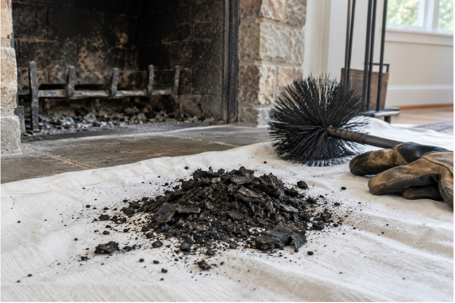
Original illustrative photo of removed deposits. Appearance alone does not establish the condition of a flue.
